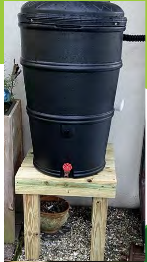
Elevating rain barrel allows gravity flow and also room to put a watering container under the spout.
