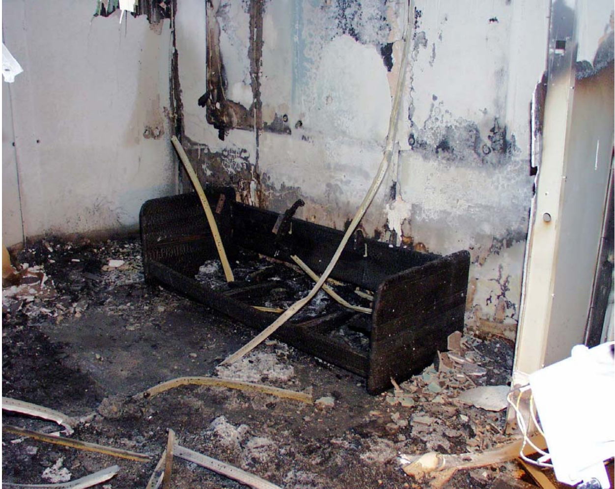
Figure 14. Photograph showing the ignition sofa after experiment 3.
