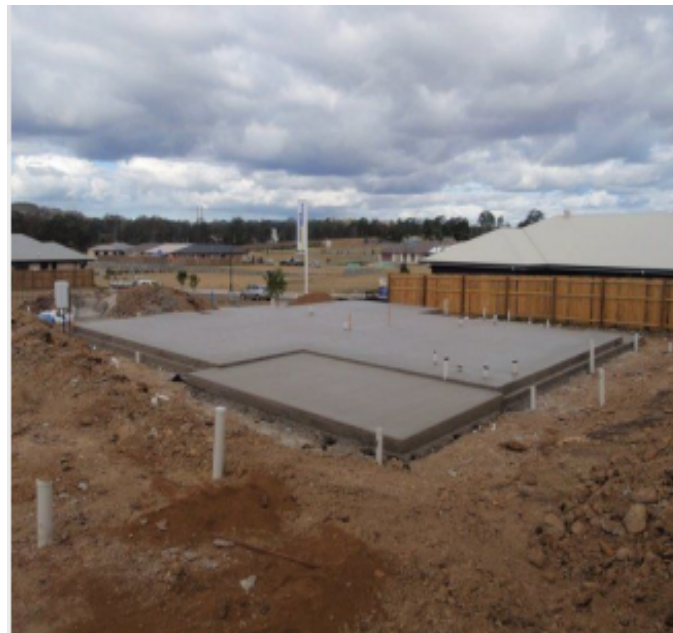
Figure 2.2.7b Slab on Grade Foundation Type
