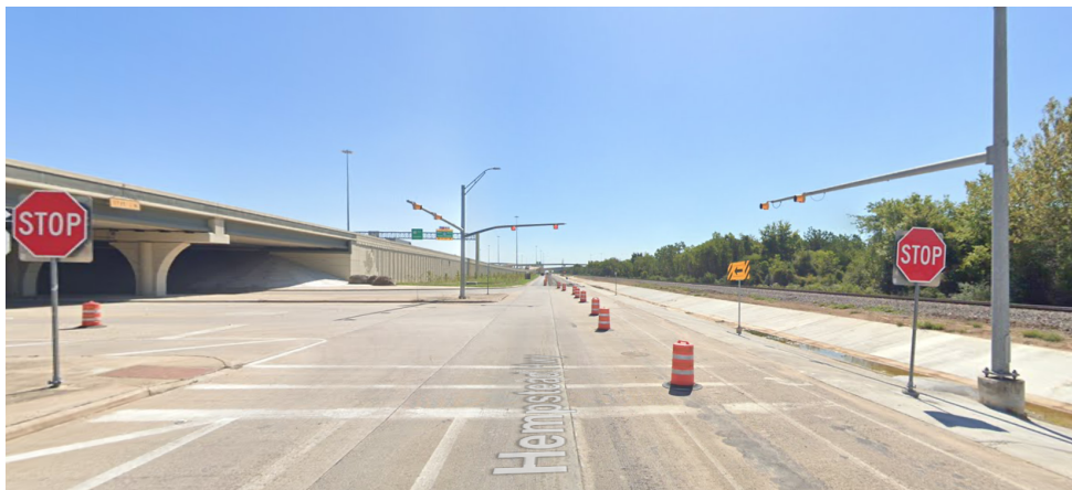
Figure 2.3.8 Gateway Blvd. & US 290 Intersection
