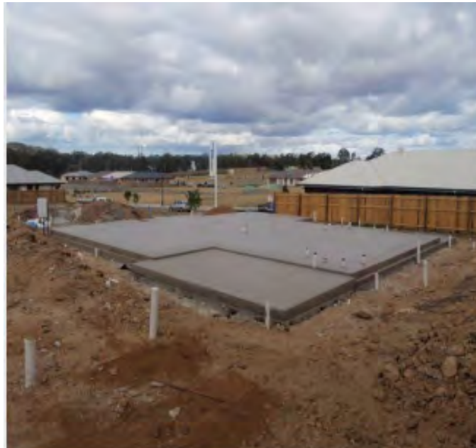
Figure 2.2.7b Slab on Grade Foundation Type
