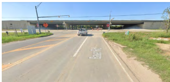
Figure 12. Existing Road Conditions
