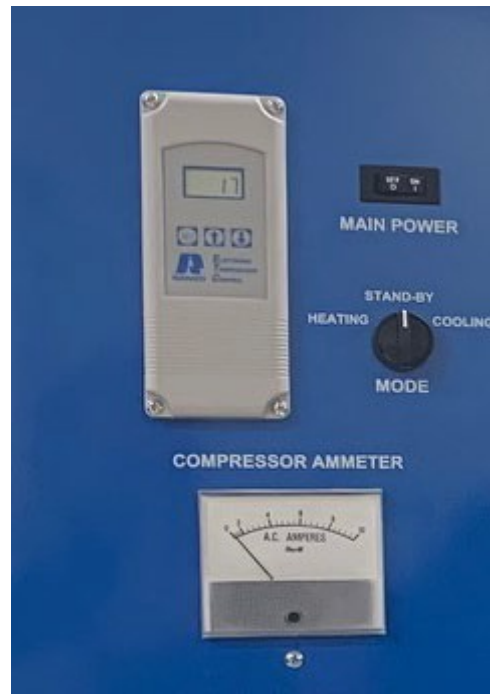
Figure 1.11 Amatrol T7082 Electronic Temperature Control
