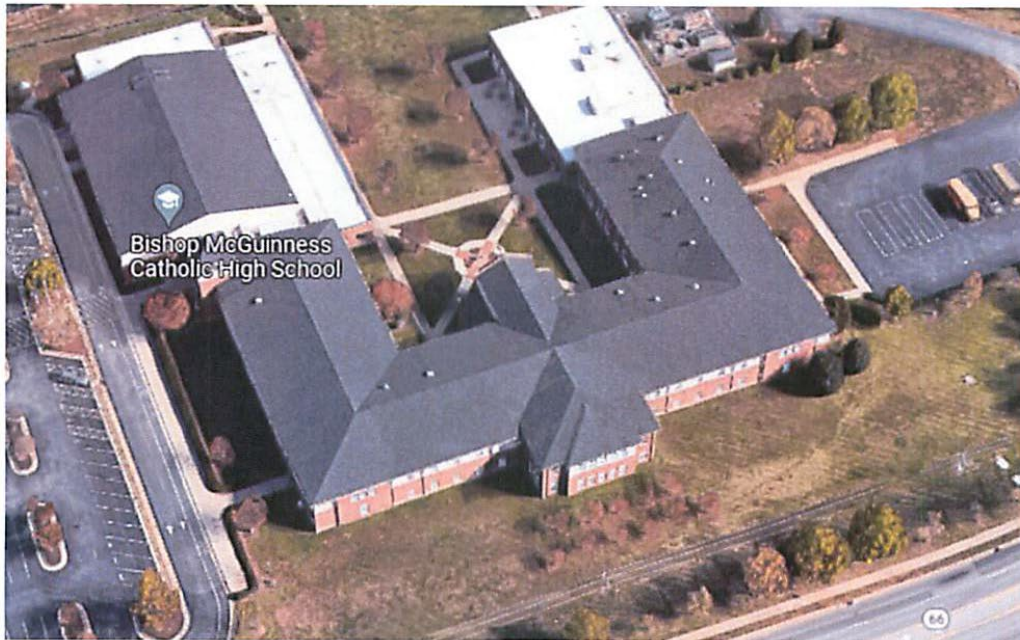
Figure 01: Existing 75,000 ft 2 building that is to be demoed
