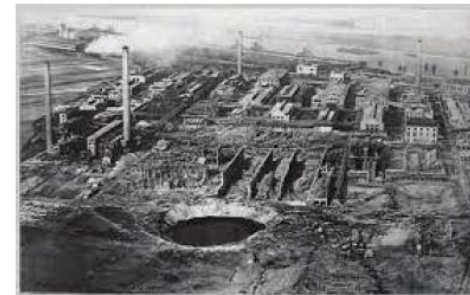
Figure 1: Photograph of the aftermath in Oppau showing the entire chemical fertilizer factory and the crater formed at the silo days after the explosion.
