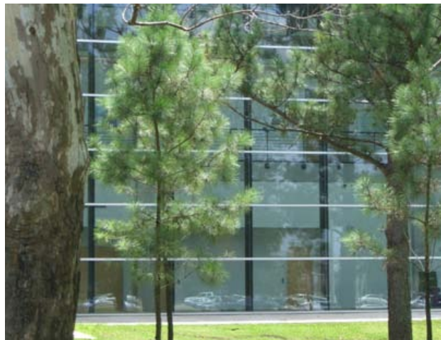
Figure 2.6: Electrical Engineering Building - Glazing
