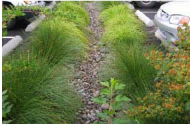
Figure 2.20: Bio-swale at parking area
