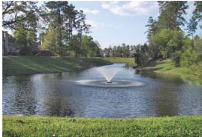
Figure 2.23: Stormwater retention pond
